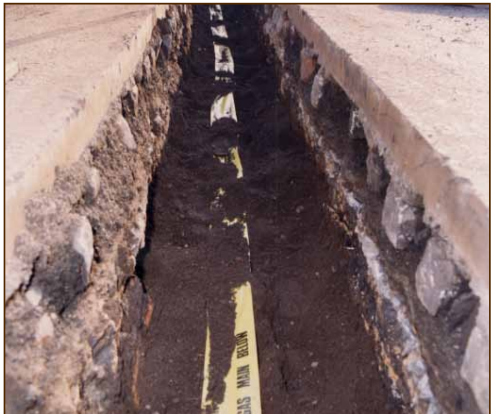
Figure 9 Yellow plastic tape, laid above a gas pipe
