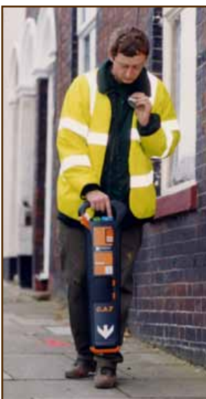
Figure 4 Using a cable locator
