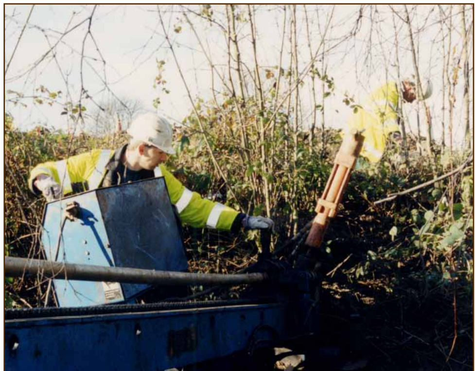
Figure 6 Horizontal drilling being used for laying a cable under a road
