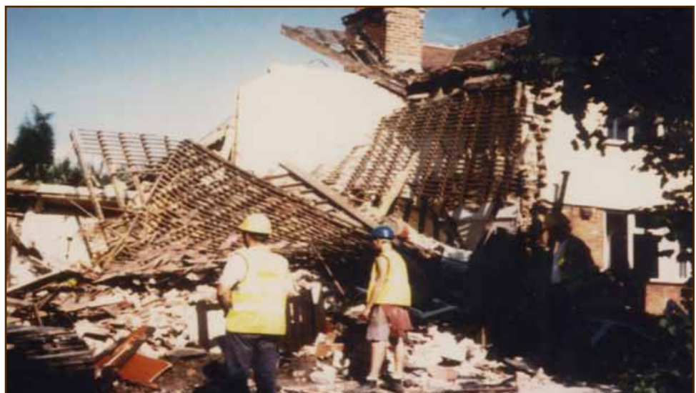
Figure 1 Aftermath of a gas explosion, following damage to an underground gas service pipe
