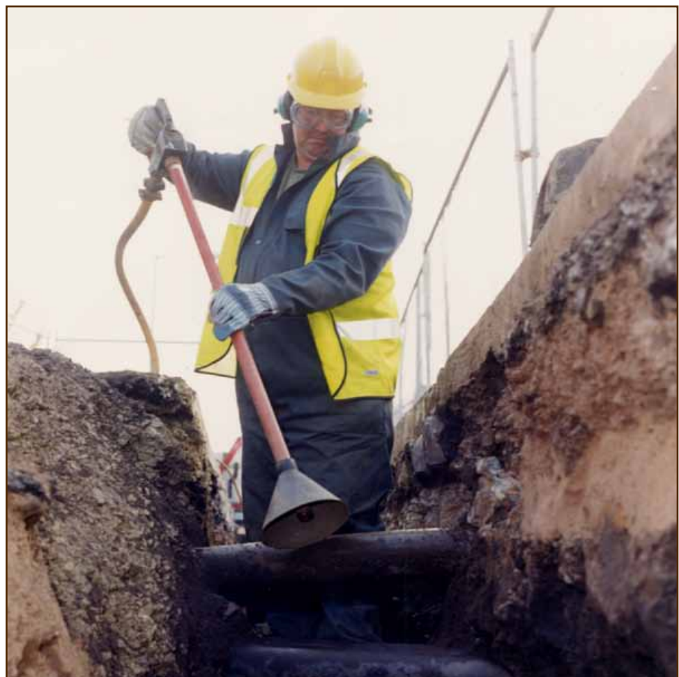
Figure 5 Using an air digging tool
