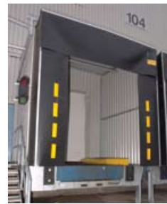
Figure 33 A well-organised loading bay, using traffic lights to inform drivers, and using visibility marking effectively
