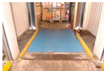
Figure 31 An extended dock leveller linking a loading bay to a vehicle load body
