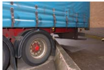
Figure 32 This concrete wheel stop helps make sure vehicles do not drive into a pedestrian area
