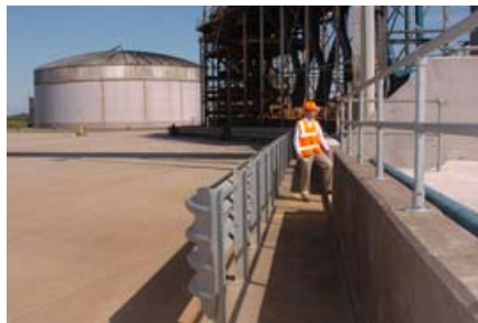
Figure 16 Barrier to protect pedestrians
