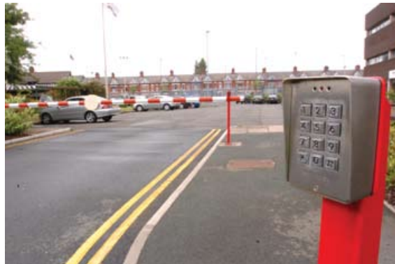
Figure 2 Key pad accessible from driving position
