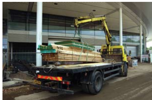
Figure 49 Vehicle unloading from firm and level ground
